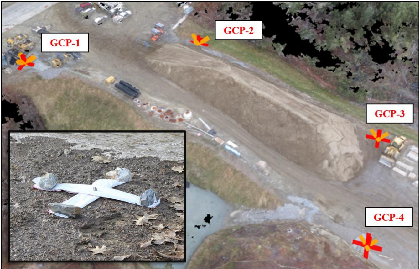
Figure 5: GCP locations in relation to stockpile
