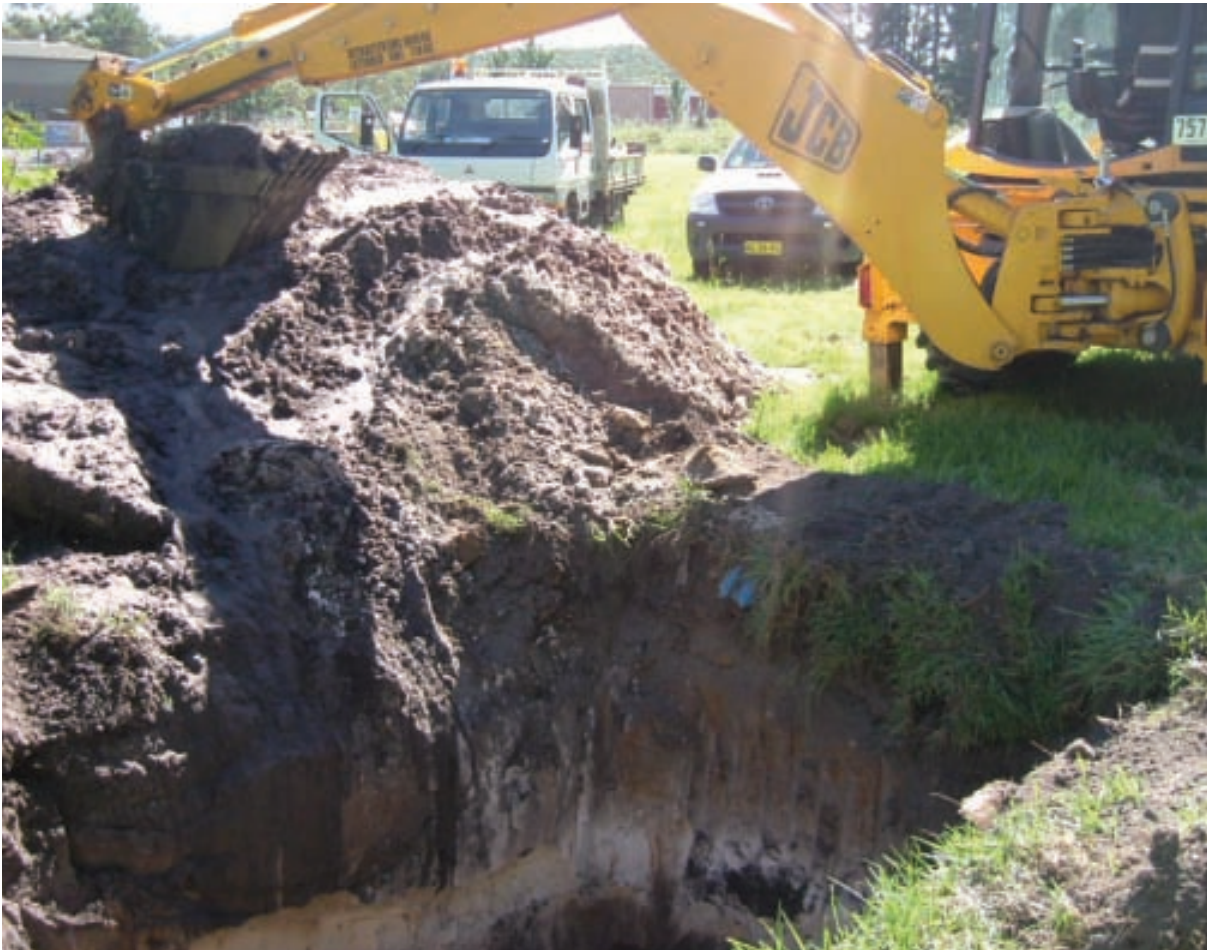
In-ground pits can be used to bury contaminated soil. Photo: Terry Inkson
