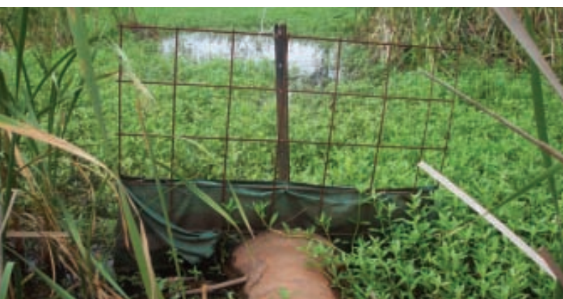
Screen made from reinforcement mesh and shadecloth.
