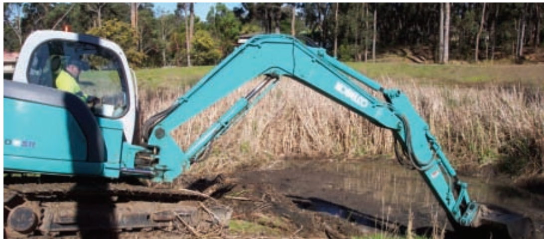
Careful shallow excavation should result in a clean, bare surface. Photo: Graham Prichard
