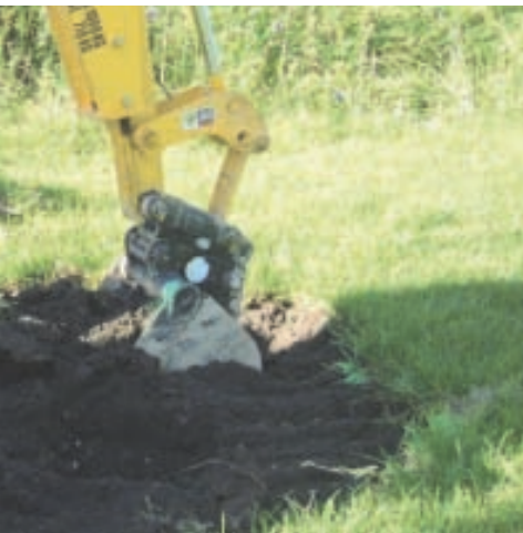
The initial scrape should be shallow. Photo: Terry Inkson
