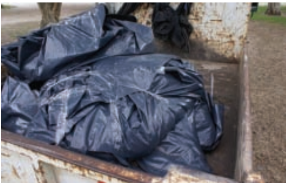
Contaminated soil can be wrapped in triple-layered black plastic before burial. Photo: Terry Inkson
