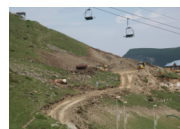
Excavation works in the French Pyrenees : soil stripping Photo : CBPS, Malaval
