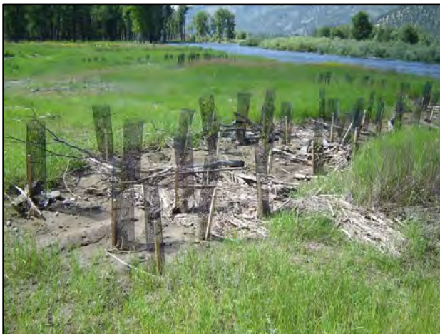
Figure 6. Constructed floodplain swales that have trapped debris and fine sediment transported during a flood event. Swale features also trap seeds and other plant propagules and provide microsites for installed container plants and natural recruitment.
