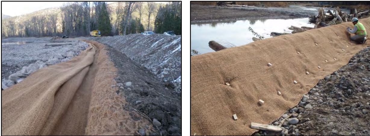
Figure 12. Construction of a wrapped coir log.
