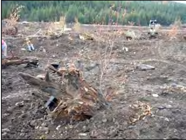
Figure 7. Large and coarse wood that is partially buried in floodplain swales creates protected microsites for planted and seeded shrubs, trees, forbs, and grasses to establish and grow.
