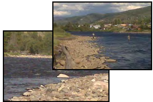
Views of the completed Phase 1 project.
