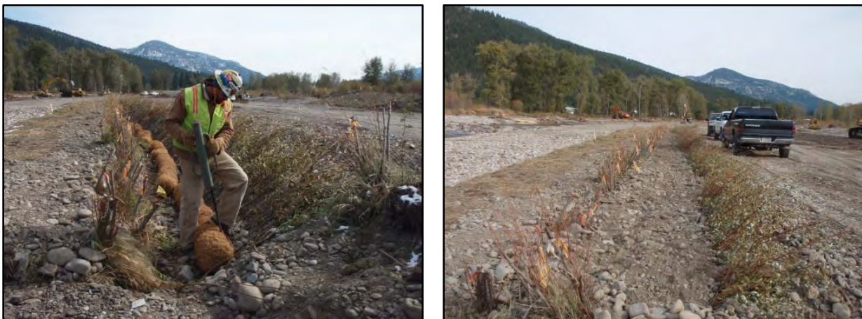
Figure 13. Construction of a vegetated brush trench.
