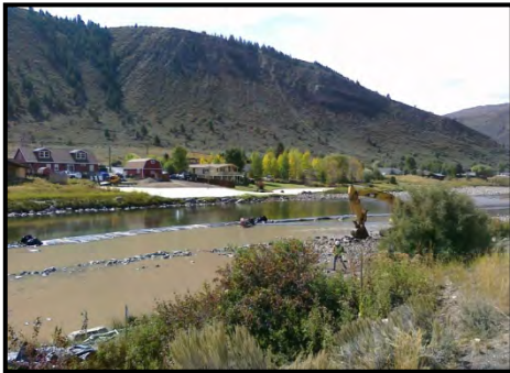
Aqua Dams functioning to contain sediments stirred up by construction
