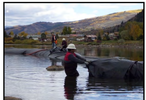
Aqua Dam installation is labor intensive.
