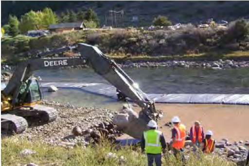
Protecting the river during construction.
