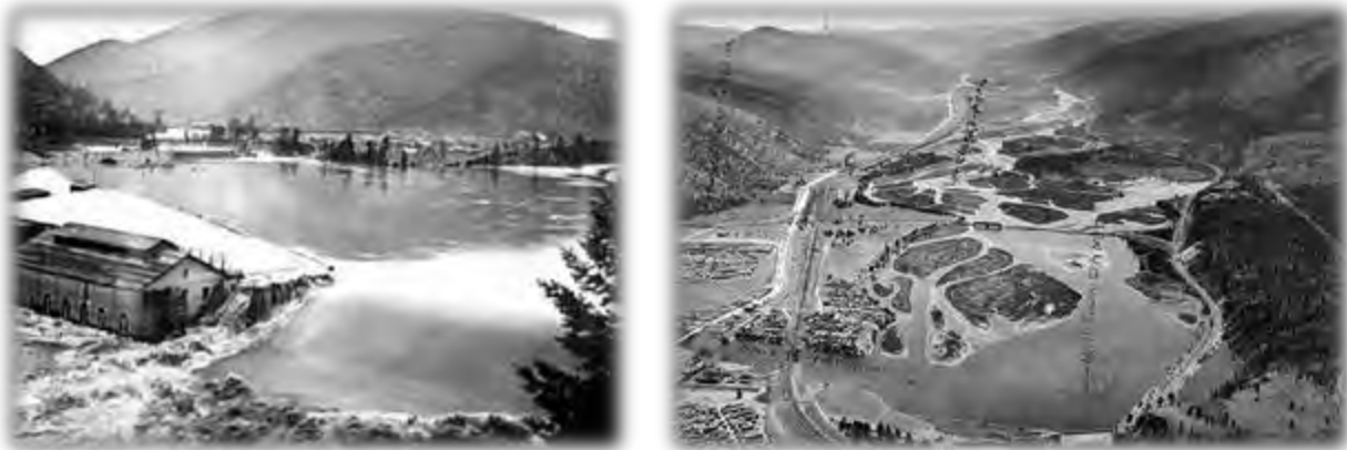
Figure 1. 1908 flood photograph at left, 1935 flood photograph on right.
