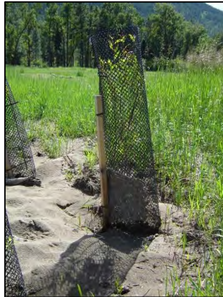
Figure 6. Constructed floodplain swales that have trapped debris and fine sediment transported during a flood event. Swale features also trap seeds and other plant propagules and provide microsites for installed container plants and natural recruitment.
