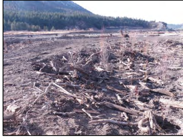
Figure 5. Large constructed floodplain swales serve as planting islands. The left photo shows a swale after excavation. The right photo shows a swale after large and coarse woody has been added and the surface has been roughened to create microsites for plants to establish.
