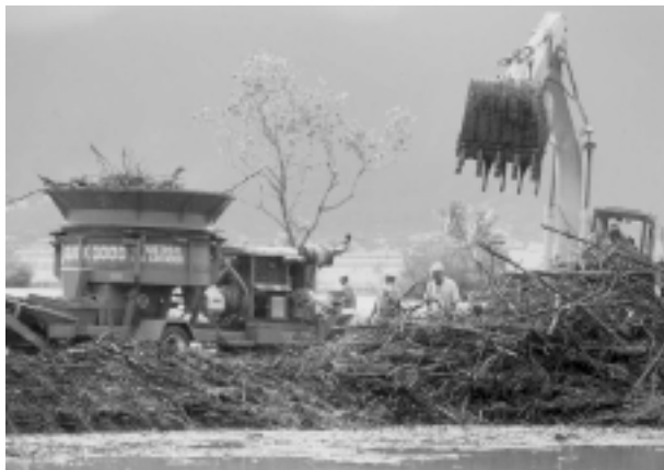
Fig. 4 Mangrove removal using heavy equipment, tub grinder and grappling arm.
