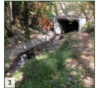
1-3 Time series of improvements in stream connectivity showing 1) old, small steel culvert 2) excavation to remove the culvert and 3) upgraded concrete box culvert in Lyall Creek, Gulf Islands National Park of Canada (British Columbia)
