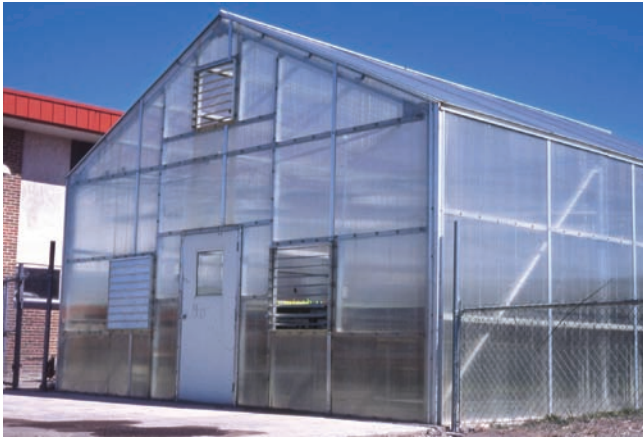
Figure 1.11 —Good site assessment and an understanding of your crop’s needs will help you determine the best structures for your nursery. Shown here is the greenhouse at the Browning High School on the Blackfeet Reservation in Montana. Photo by Tara Luna.
