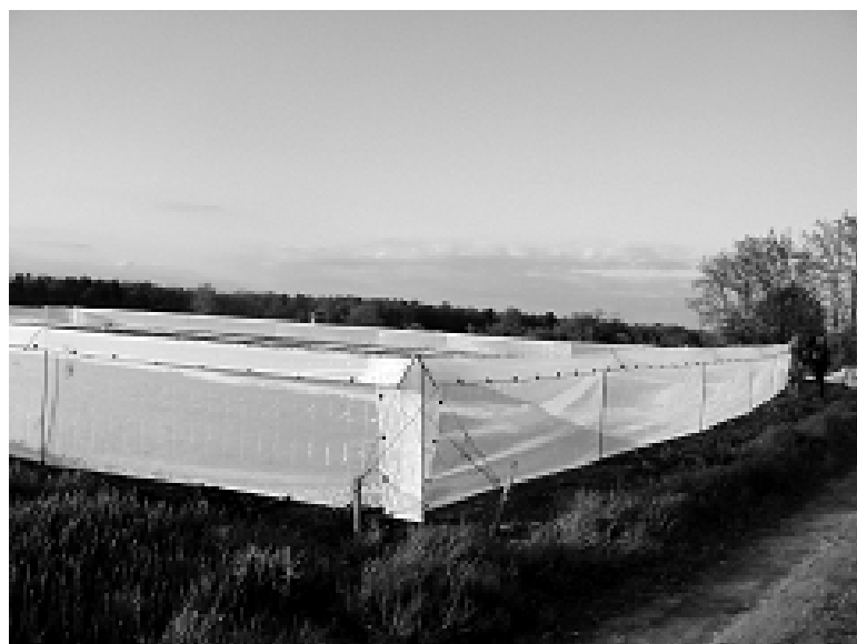
Photo 1: Construction du FiBL-INSECTSTOP (Photo Winterling 2005).
